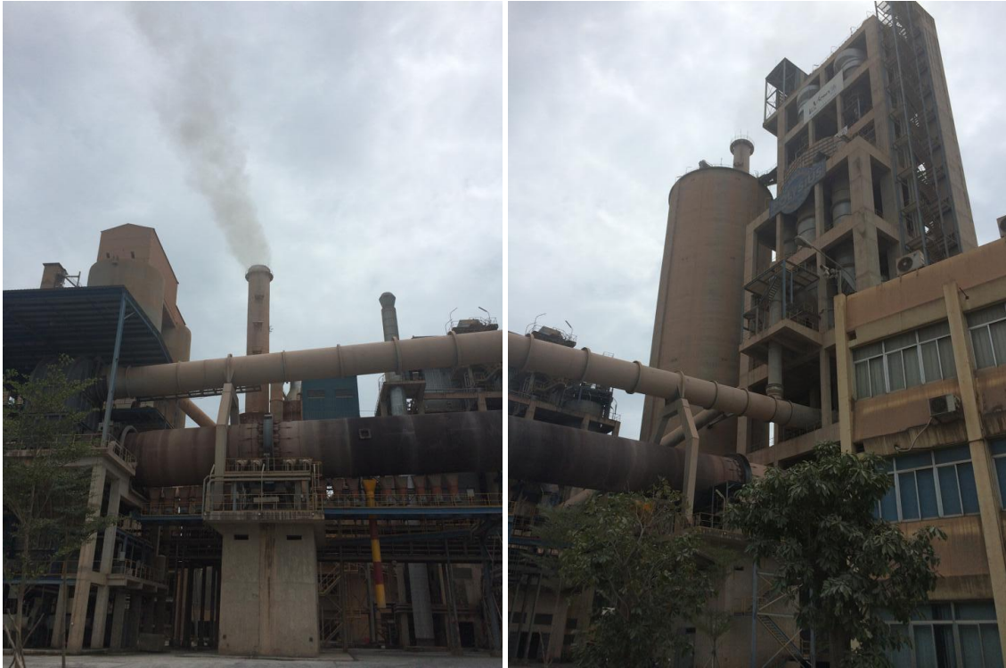
Figure 2: The kiln and preheater in Ha Tien 1 cement facility in Kien Giang province.
