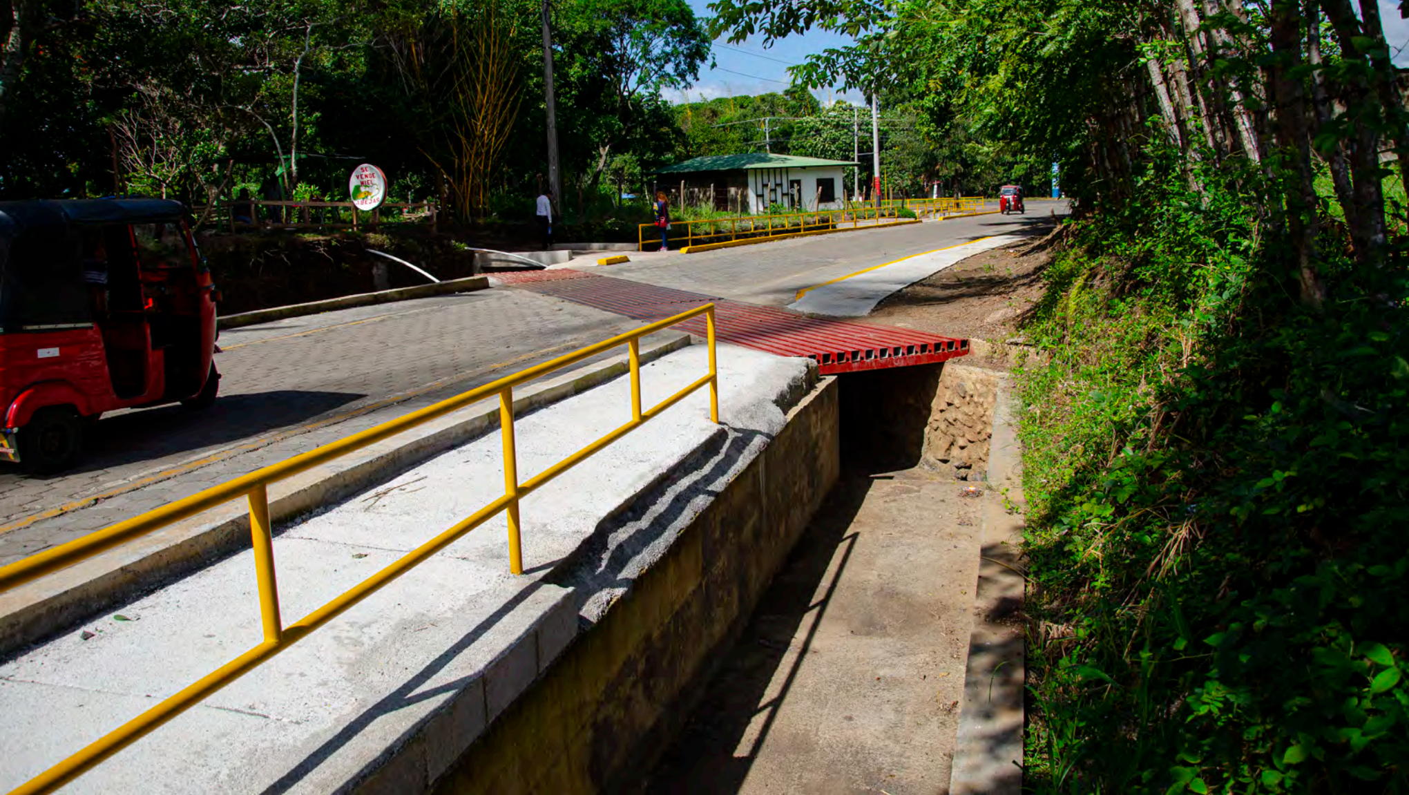
Guanacaste pilot project, Nandaime-Granada junction. Complementary works were incorporated to protect pedestrians and access bridges to homes located on the other side of the channel.
