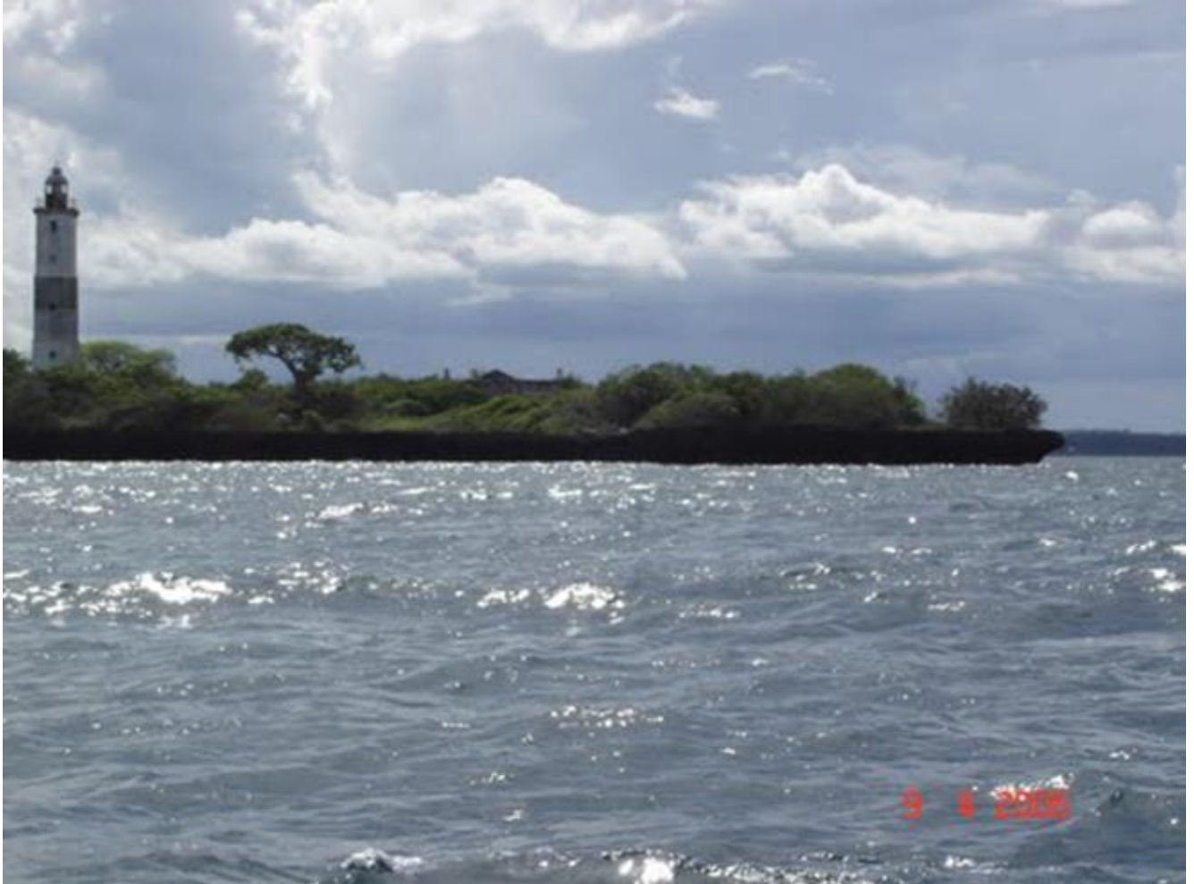
Figure 27: Lighthouse on Ulenge Island, north of Tanga, Photo from Google Earth
