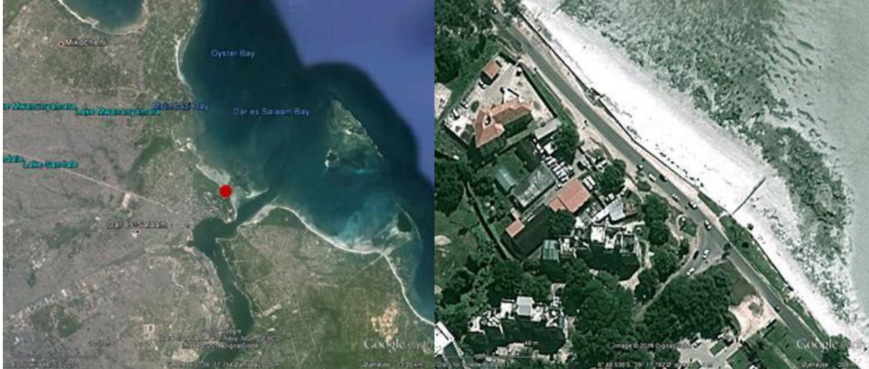
Figure 41: Example of coastal protection works in Dar es Salaam: a sea wall protecting a road close to the coastline.
